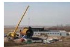
Delivering parts for the new airport fire brigade training centre
