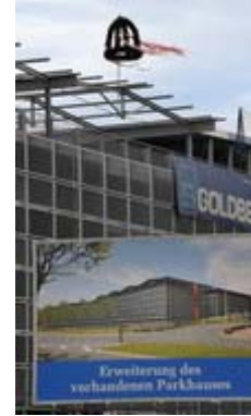
Topping-out ceremony for the car park extension on 16 March 2010
