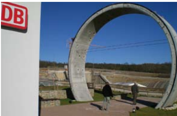
A ring of the tunnel bore rises next to the information centre – this will be its size.
