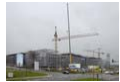
The building work in April 2010
