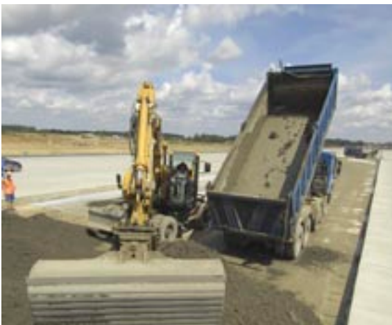
The concrete was laid along 15-metre wide strips
