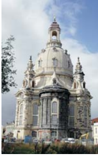
Work to rebuild the Frauenkirche started 1996
