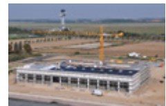
The eastern fire station is being built in Kursdorf
